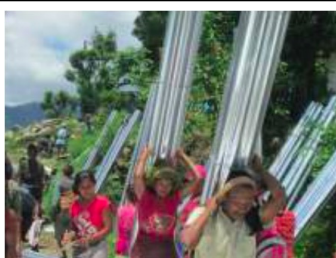
Carrying materials to site
